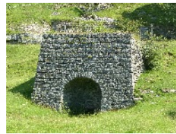
Lime kilns are a common feature of limestone areas. Limestone (calcium carbonate) was burnt to produce quicklime (calcium oxide), used in mortar and also spread on the fields to neutralise acid soils.
